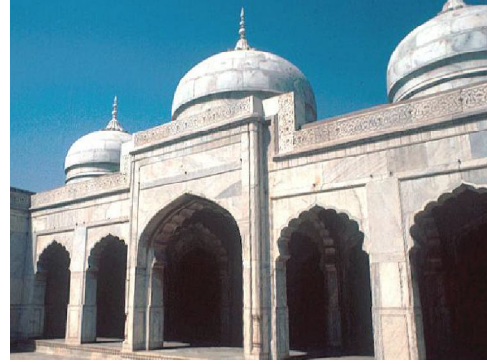
Figure 6: East Façade of Pearl Mosque, Lahore
