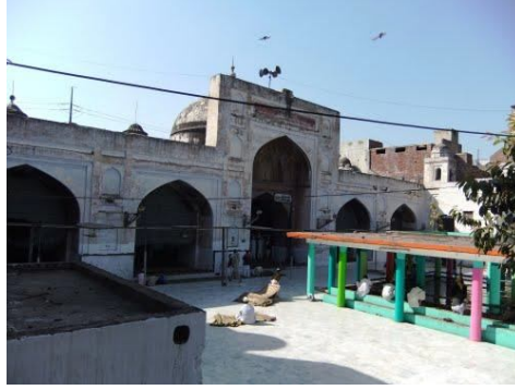
Figure 8: External View of Maryam Zamani Mosque
