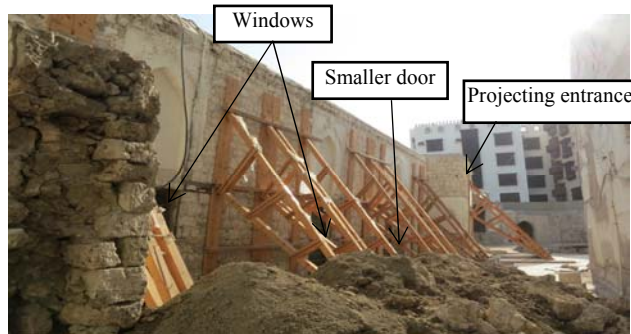
Fig. 9: Al-Shafi'i Mosque Exterior Northern Wall
