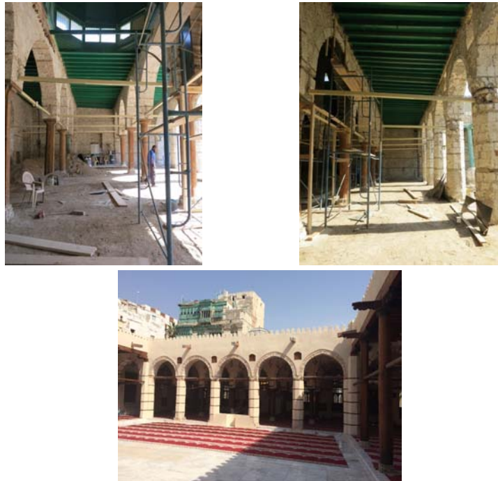
Fig. 16: Al-Shafi'i Mosque Qibla Riwaq During (Above) and (Below) After Restorations
