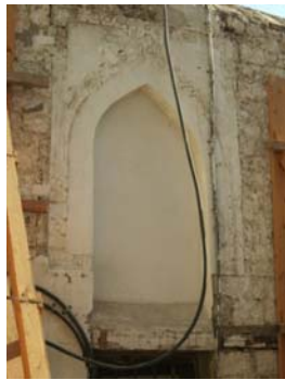
Fig. 11: Blind Pointed Arch Above the Door
