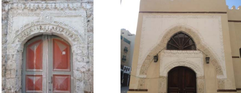
Fig. 6: Al-Shafi'i Mosque Small Door on the Southern End of the Qibla Wall, Before and After Recent Restoration
