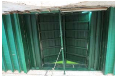
Fig. 22: Al-Shafi'i Mosque First Opening in the Ceiling
