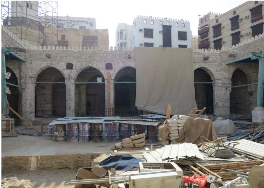
Fig. 25: Al-Shafi'i Mosque Southern Wall
