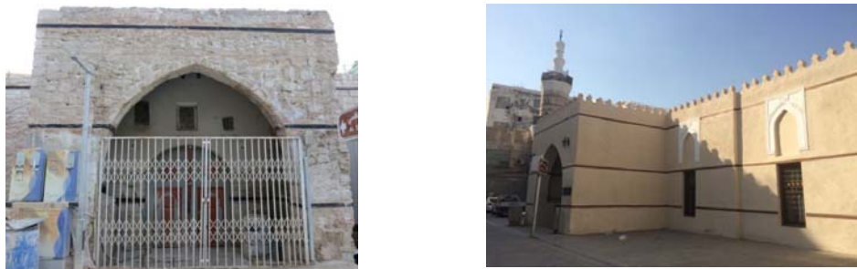
Fig. 7: Al-Shafi'i Mosque Southern Wall, Main Entrance Before and After Restoration. The Entrance's Projection is Shown in the New Picture
