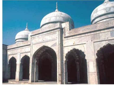
Figure 6: East Façade of Pearl Mosque, Lahore
