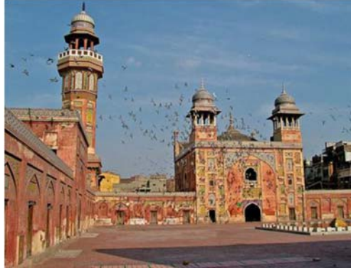
Figure 10: Wazir Khan Mosque Courtyard
