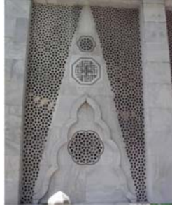
Figure 18: Façade of Masjid-e-Shohada Showing Use of Screens
