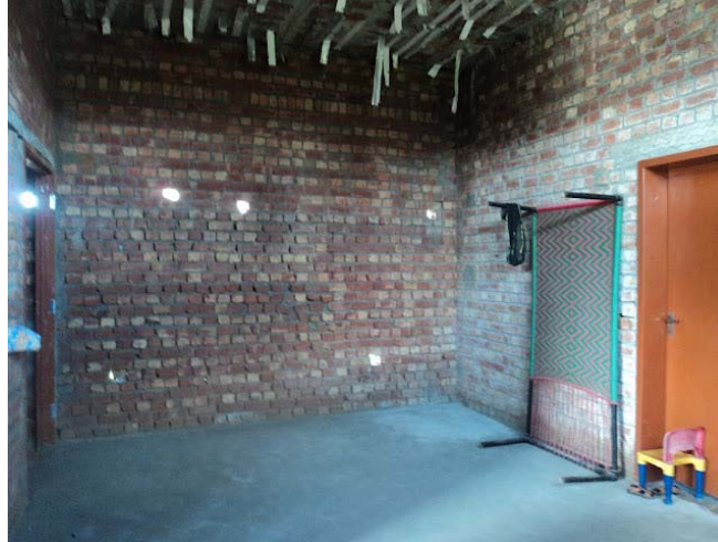
Figure10: Incremental Construction of a House Stopped Due to Non-Availability of Funds
