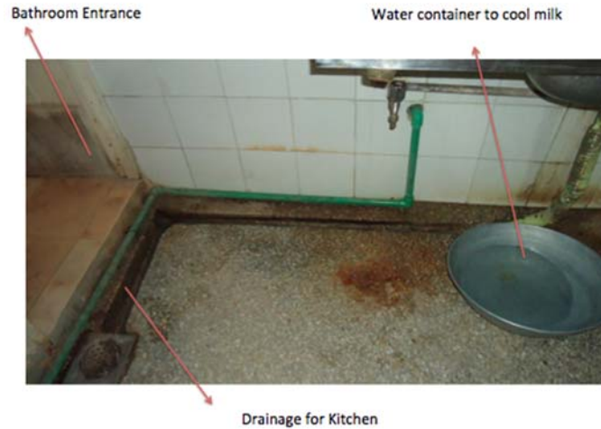
Figure 8: Bathroom Entrance, Drainage for Kitchen and Food Storage at One Place
