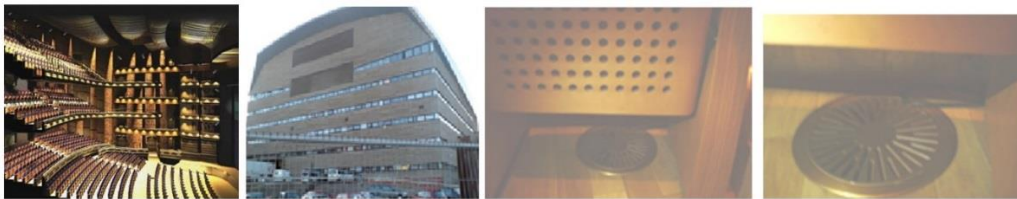
Figure 2. Internal view of main hall, external supply and extract openings, supply grills under seats, source: Author
