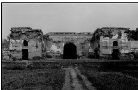
Figure 4. Jahangir's tomb destruction and encroachments
