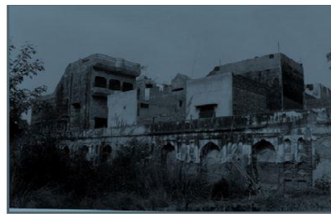
Figure 5. Encroachments along Jahangir tomb's boundary wall
