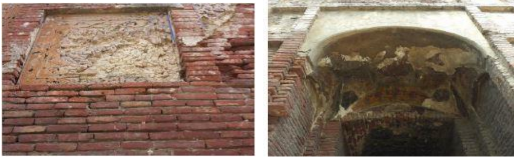
Figure 6. Nawankot Monument's decay Figure 7. Nawankot Monument ornamentation decay
