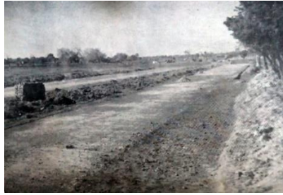
Figure 2. Preparations for construction (Source: LIT)
