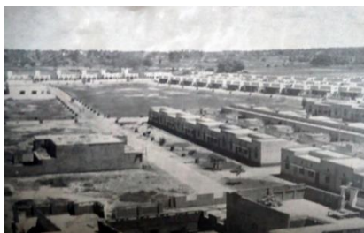
Figure 4. Samanabad Quarters Under-Construction (Source: LIT)
